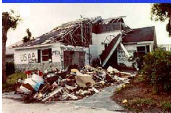
Level 3 - Major damage; uninhabitable
